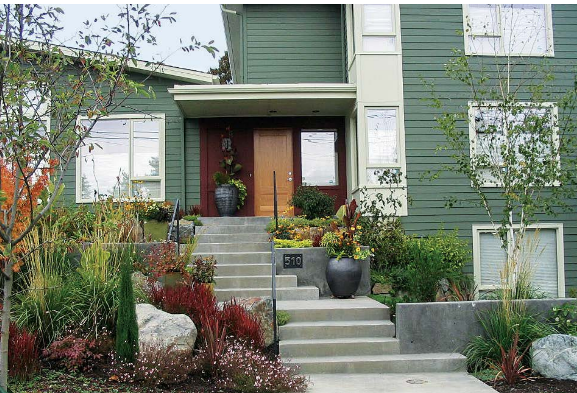
PLAN AHEAD FOR PLACES TO REST. These concrete stairs provide a handsome stepped walkway through a colorful garden. Note the location of the landings, which provide visitors with a place to catch their breath every four risers.
